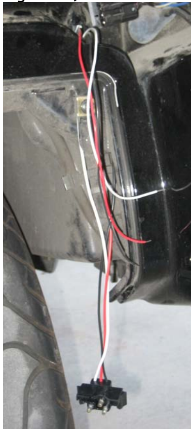
Figure 12. Wiring harness hanging loose.
