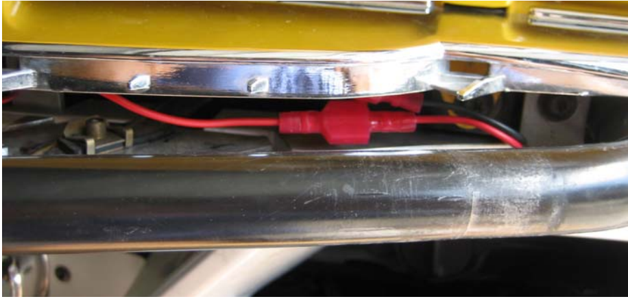
Figure 8: Wires tucked under chrome cover
