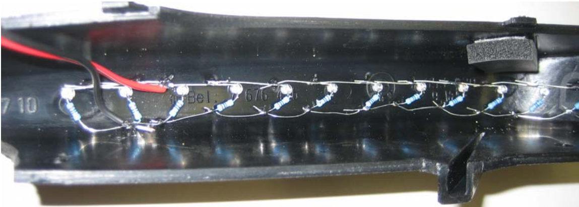
Figure 12: Close-up of zip cord attached to LEDs
