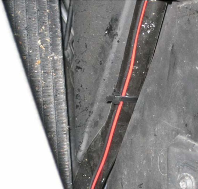
Figure 20: Zip cord secured with 7" black cable tie
