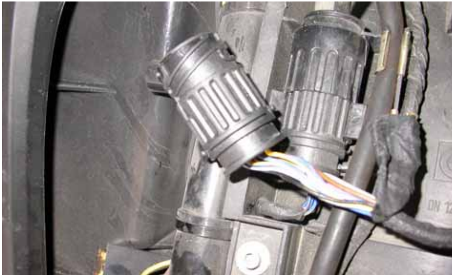
Figure 12. Wrapping cut back to expose the wires
