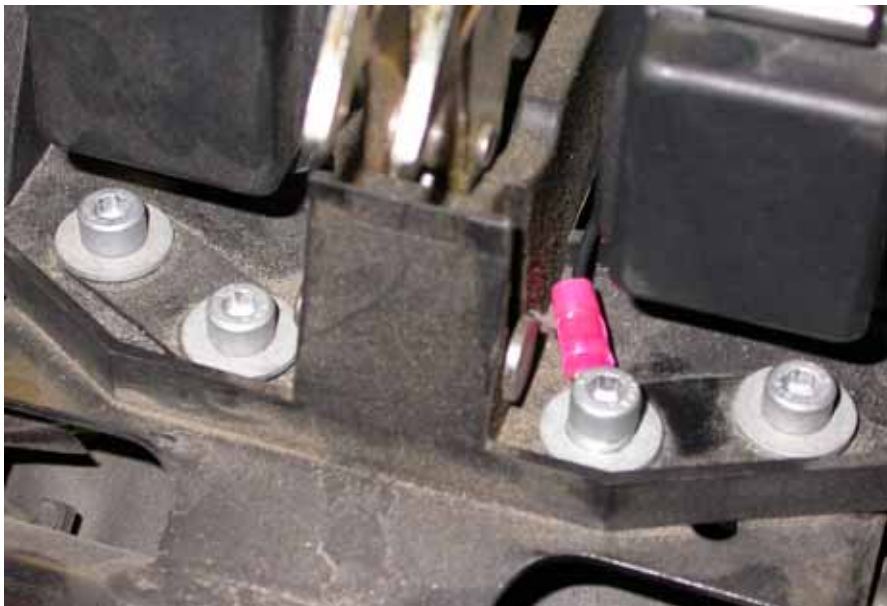
Figure 19. Ground wire connected
