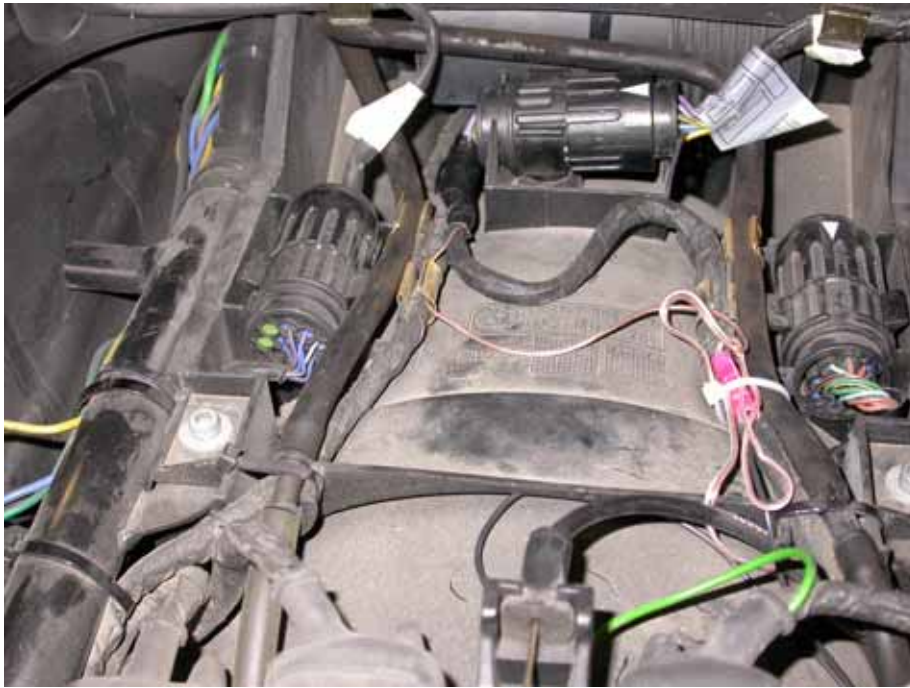
Figure 21. Wires routed and secured with cable tie for one light (viewed looking back from driver's seat)
