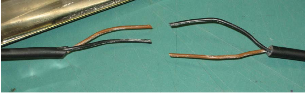
Figure 7. Insulation trimmed and wires cut
