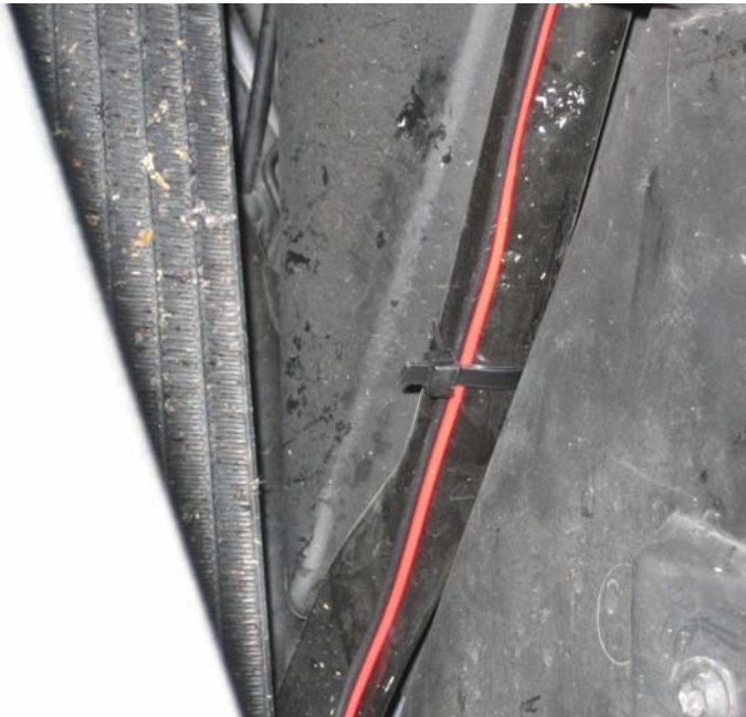
Figure 17: Zip cord secured with 7" black cable tie.
